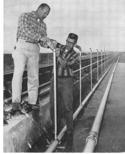
RAIN SYSTEM at the Holloman rocket sled track stretches for 6000 ft. on both sides of the track. Bill Farmer, left, and Don Hansen work on the system which creates the rainfall.
